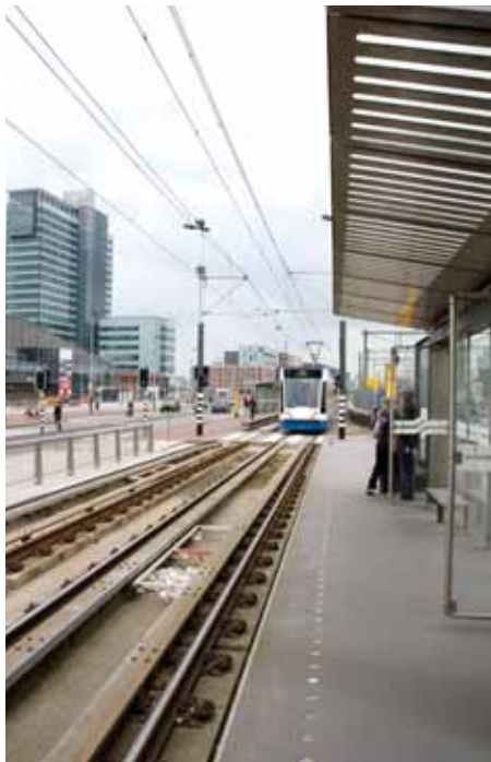
Amsterdam builds tram links before putting up new housing Photo: Els Dekker
