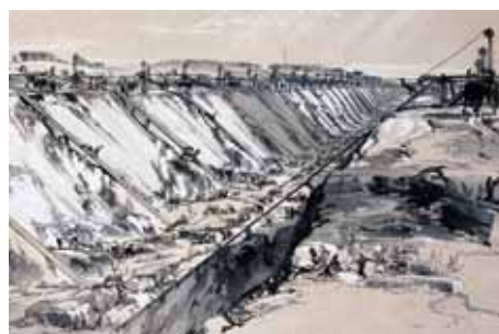
The method of excavating deep cuttings like at Primrose Hill
